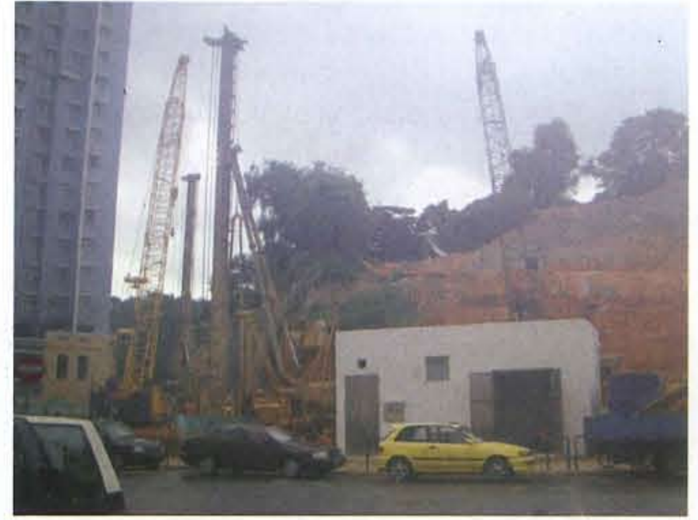
Bulroc's CDS system is designed to produce straight piles
